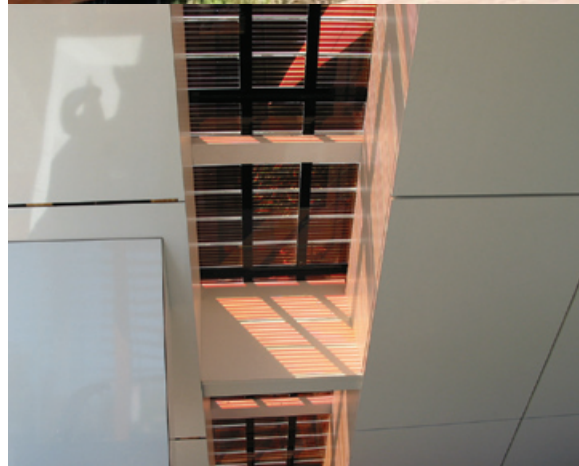
House of the future, Sydney Olympic Park
