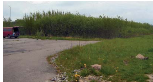
Phytoremediation of a former gas-station in Rønnede (Denmark) using different species of Salix .
