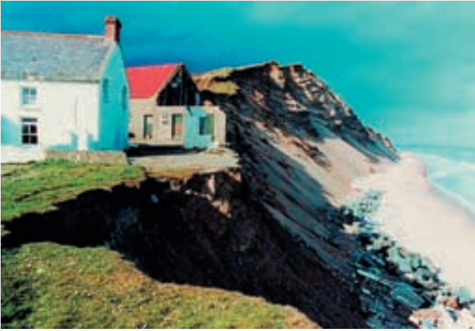
Coastal erosion. © Marine Institute, Ireland
