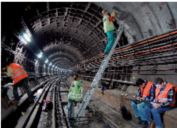
Field Trials at tunnels in Prague metro
