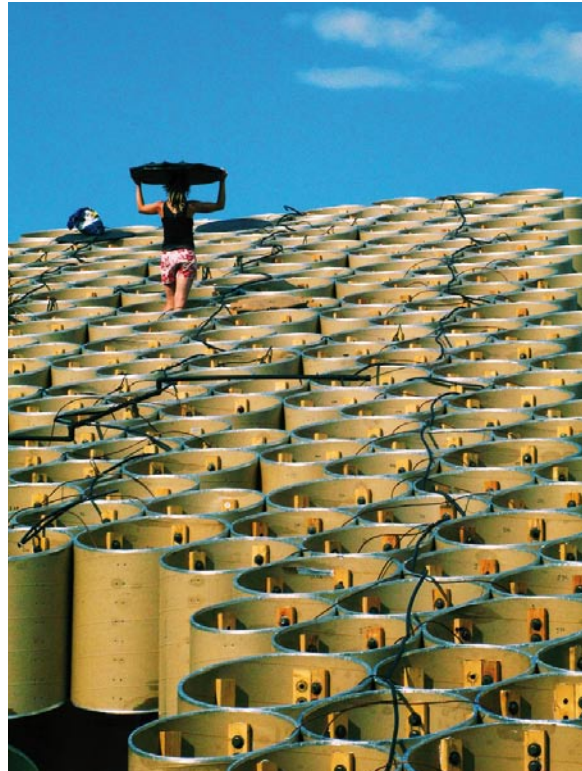
Figure 17. Modern plantation by Taís Melillo. This photograph depicts the Public Farm One (P.F.1) by WORK Architecture Company from New York, who won the ninth annual MoMA/P.S.1 Young Architects Program in 2008 with this urban farm concept. Constructed from large cardboard tubes, the top surfaces of P.F.1 act as a working farm, nowadays blooming with a variety of vegetables and plants. P.F.1 is conceived as a living structure made from inexpensive and sustainable materials, an interactive bridge between outside and inside space with multiple zones of activity.
