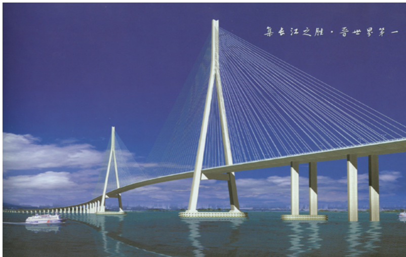
Sutong Bridge, Jiangsu, China
