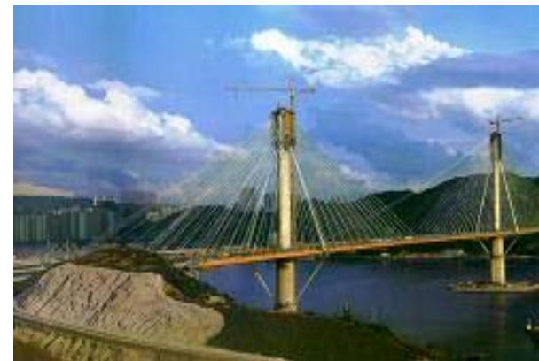
Ting Kau Bridge
