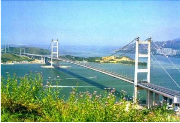
Tsing Ma Bridge
