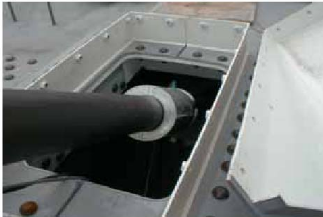
Sensor Beneath the Deck
