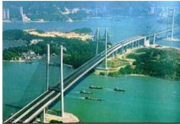
Kap Shui Mun Bridge
