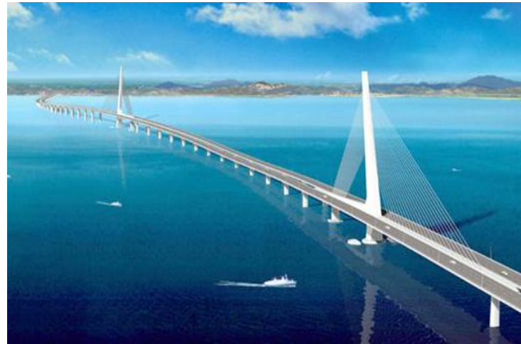
Shenzhen Western Corridor
