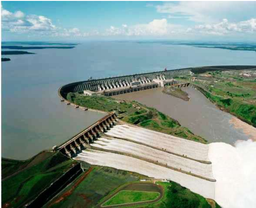
Itaipú dam (BR-PY)
