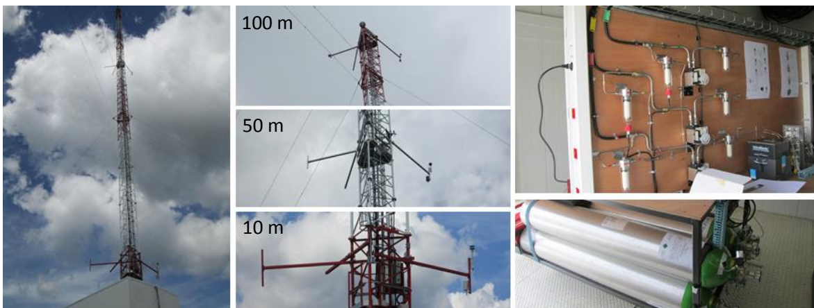
Fig.3. ICOS tower and infrastructure for measurements of atmospheric concentrations of greenhouse gases at three levels (10, 50 and 100 m) at Observatoire de Haute-Provence, France
